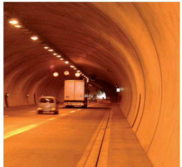
Road tunnels provide direct connections and are indispensable for efficient road networks (source: BAST)
